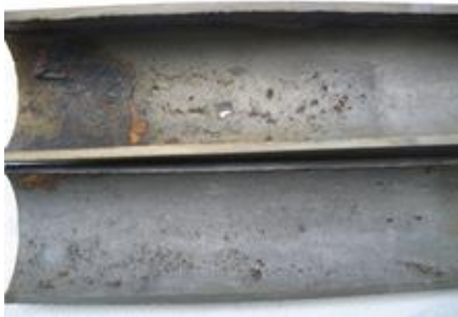
Internal storage-corrosion example
